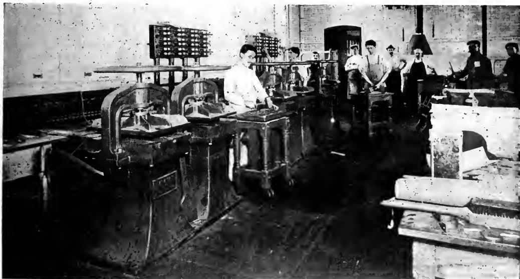
FIG. 28.—ELECTRIC HEATING DEPARTMENT. FIRST ELECTRICALLY-HEATED MATRIX PRESSES EVER MADE.
